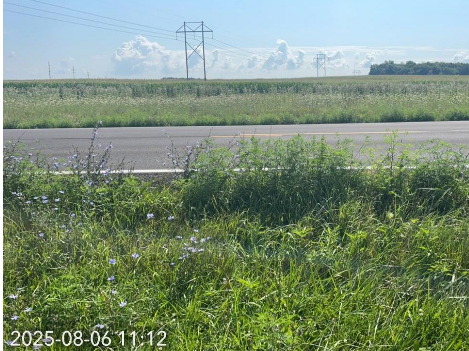
Photo Location 3. Representative view of existing road within the Project area. Photograph taken facing east.
