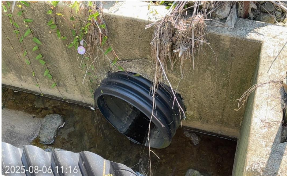
Photo Location 6. Representative view of existing culvert. Photograph taken facing east.
