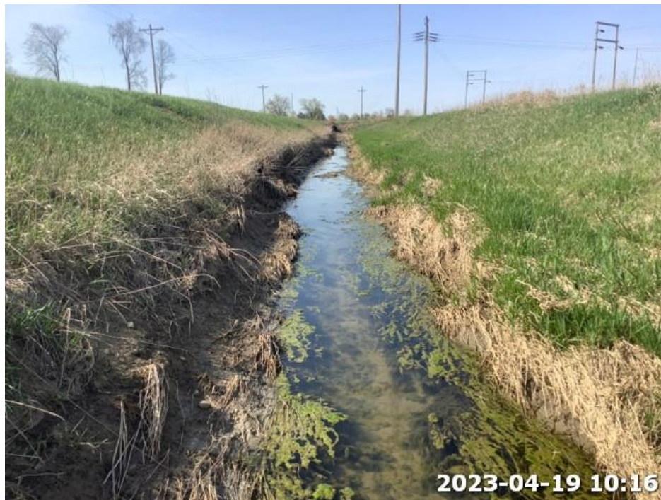
Photo Location 4. View of Stream 1. Photograph taken facing downstream/south.
